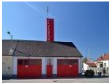
Image 19. Fire station - source: wiki commons, Herzi Pinki
