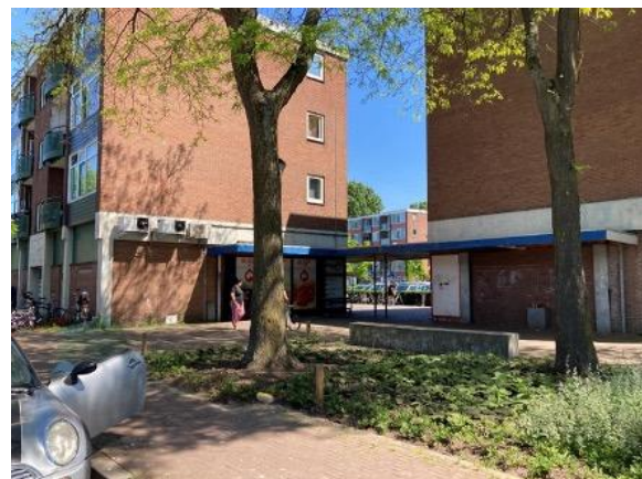
Image 11. Deltabuurt maintenance issues
